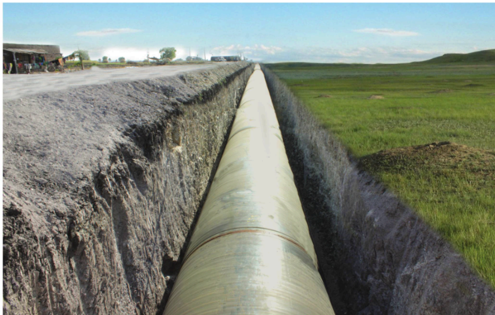
Bulk water supply: 3000 MM diameter pipeline (Gujarat)
