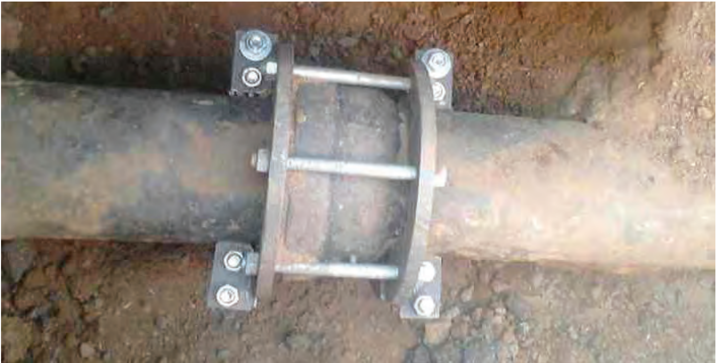
Mechanical joint in supply pipeline in Bengaluru NRW Project
