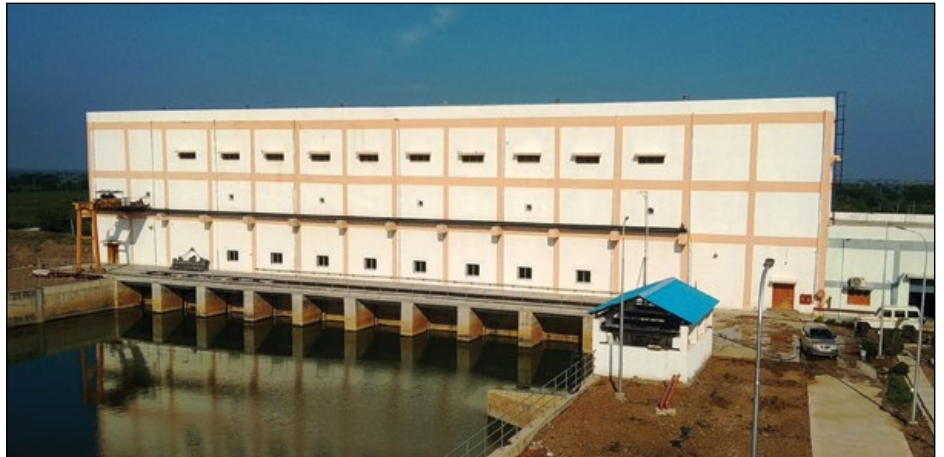
2587 MLD Pumping House for SAUNI Yojana Phase-1, Gujarat
