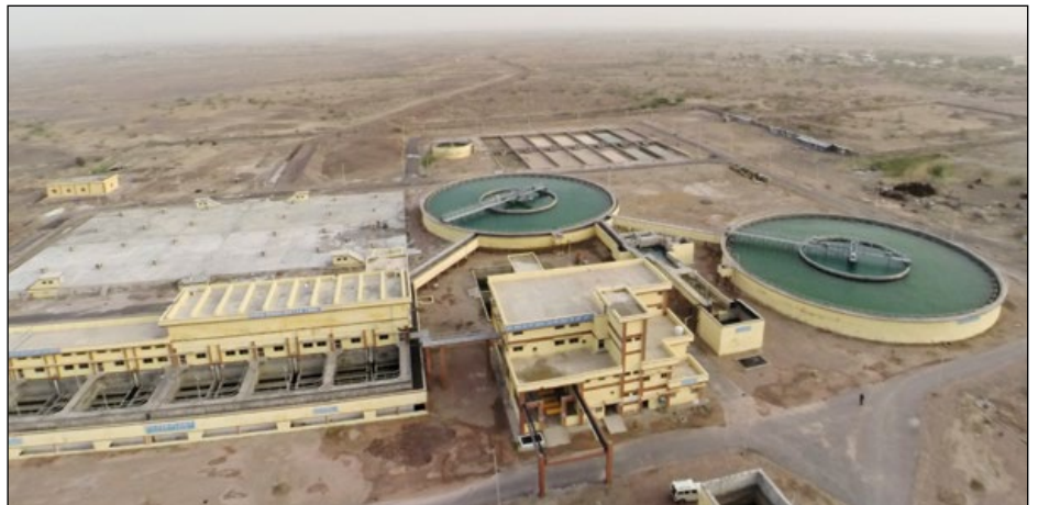
Aerial View of Pokhran Water Supply Project
