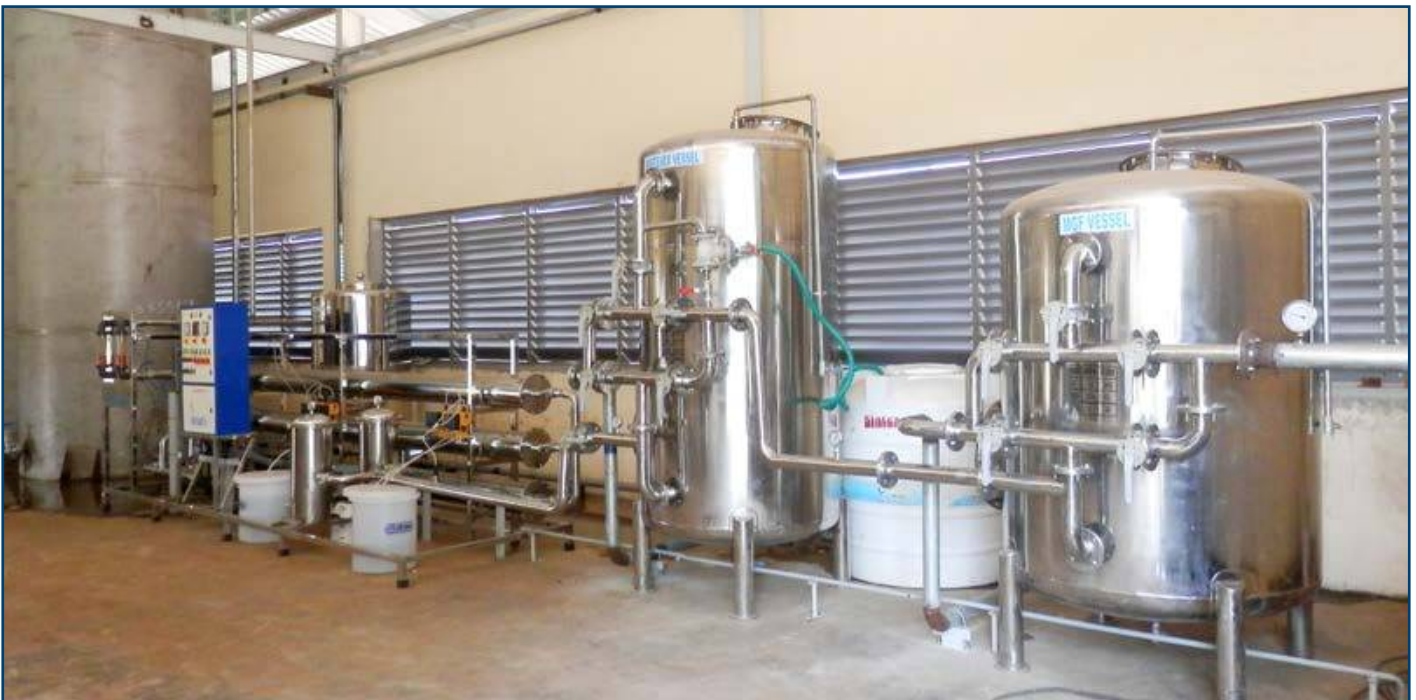
600 KLD Reverse Osmosis System for Boiler Feed
