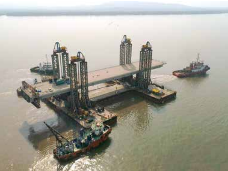
▲ Tata Projects along with partner launched a huge 90-metre-long orthotropic steel deck for the MTHL project.
