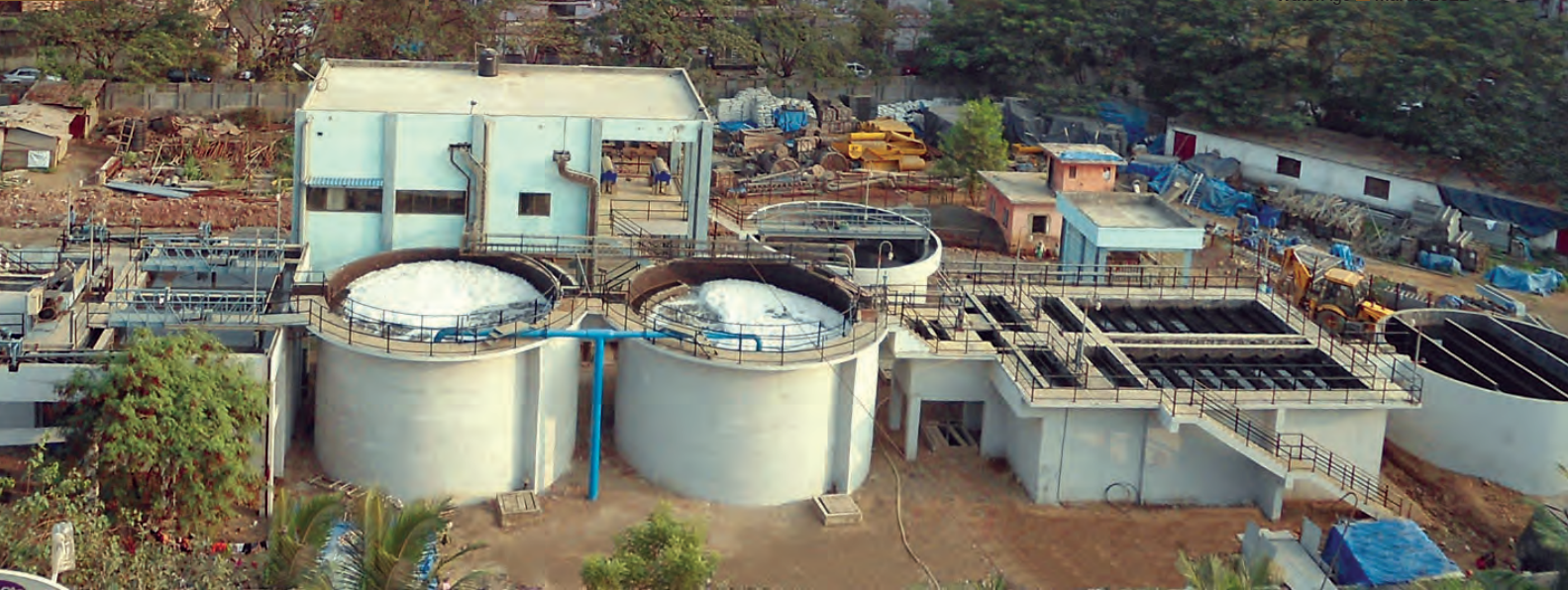
11 MLD Decentralised Sewage Treatment Plant at Mira Bhayander
