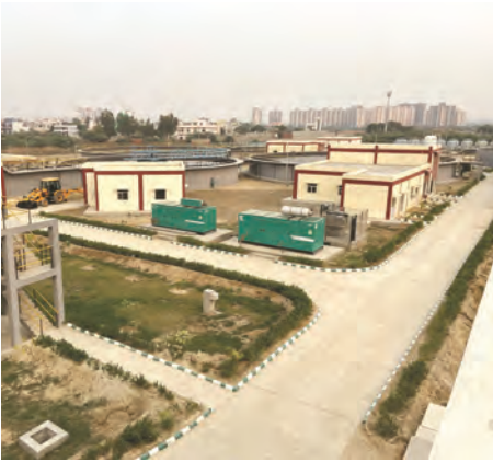
12.5 MLD Effluent Treatment Plant, Bahadurgarh Industrial Area, Haryana
