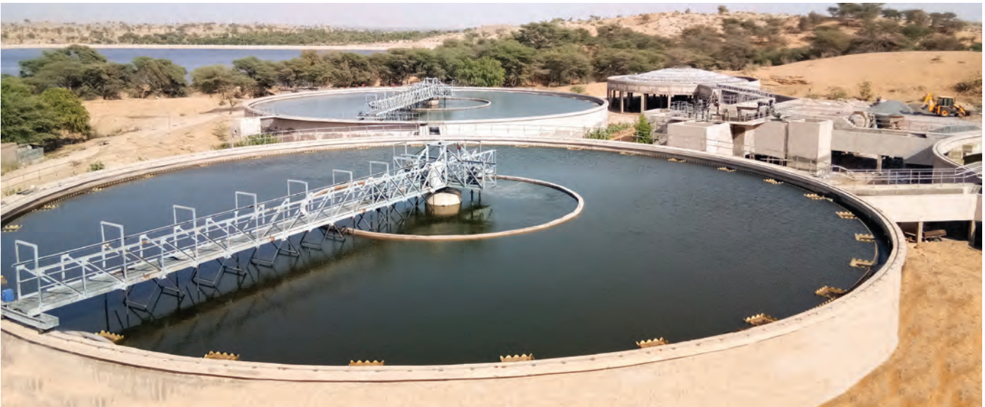
160 MLD Water Treatment Plant, Dhannaser, Rajasthan
