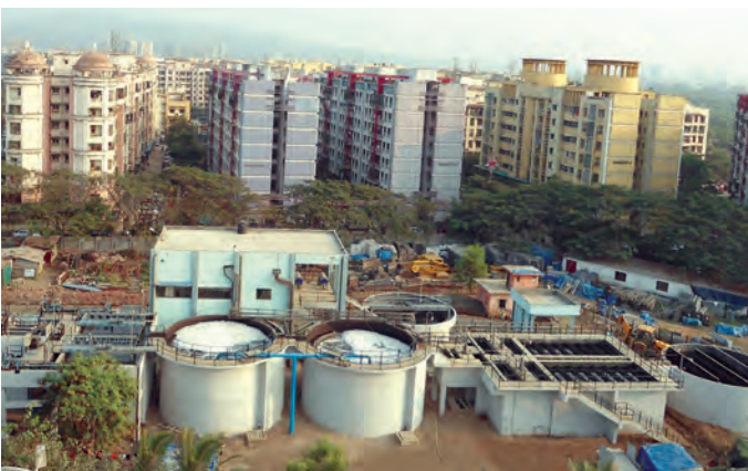
11 MLD Decentralised Sewage Treatment Plant at Mira Bhayander
