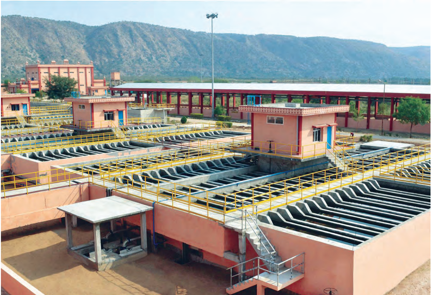
200 MLD Water Treatment Plant, Surajpura, Rajasthan
