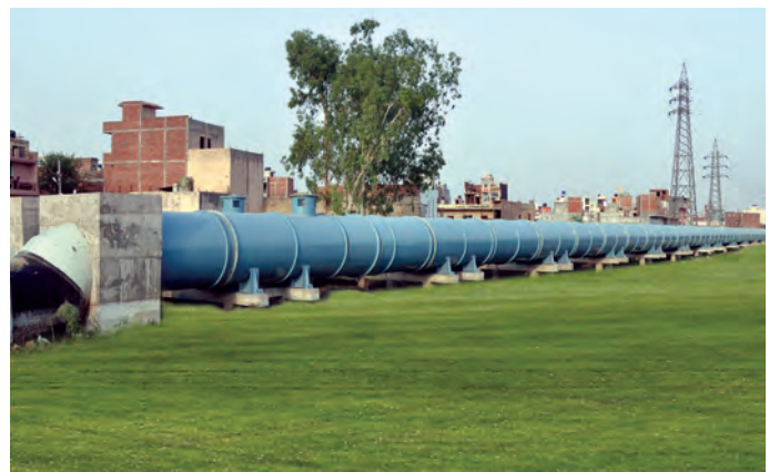
2420 MM MS Pipeline for Bulk Water Supply in Delhi
