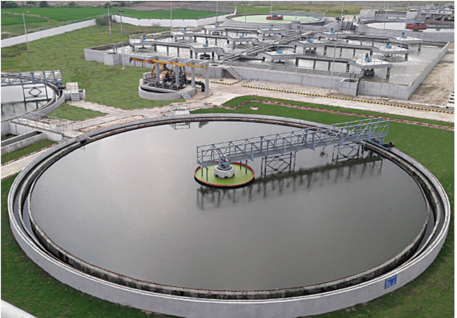
42 MLD Sewage Treatment Plant, Kanpur
