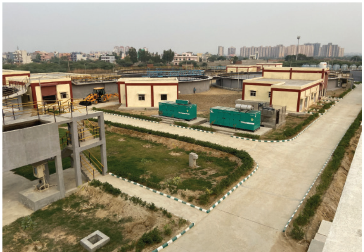
12.5 MLD Effluent Treatment Plant, Bahadurgarh Industrial Area, Haryana
