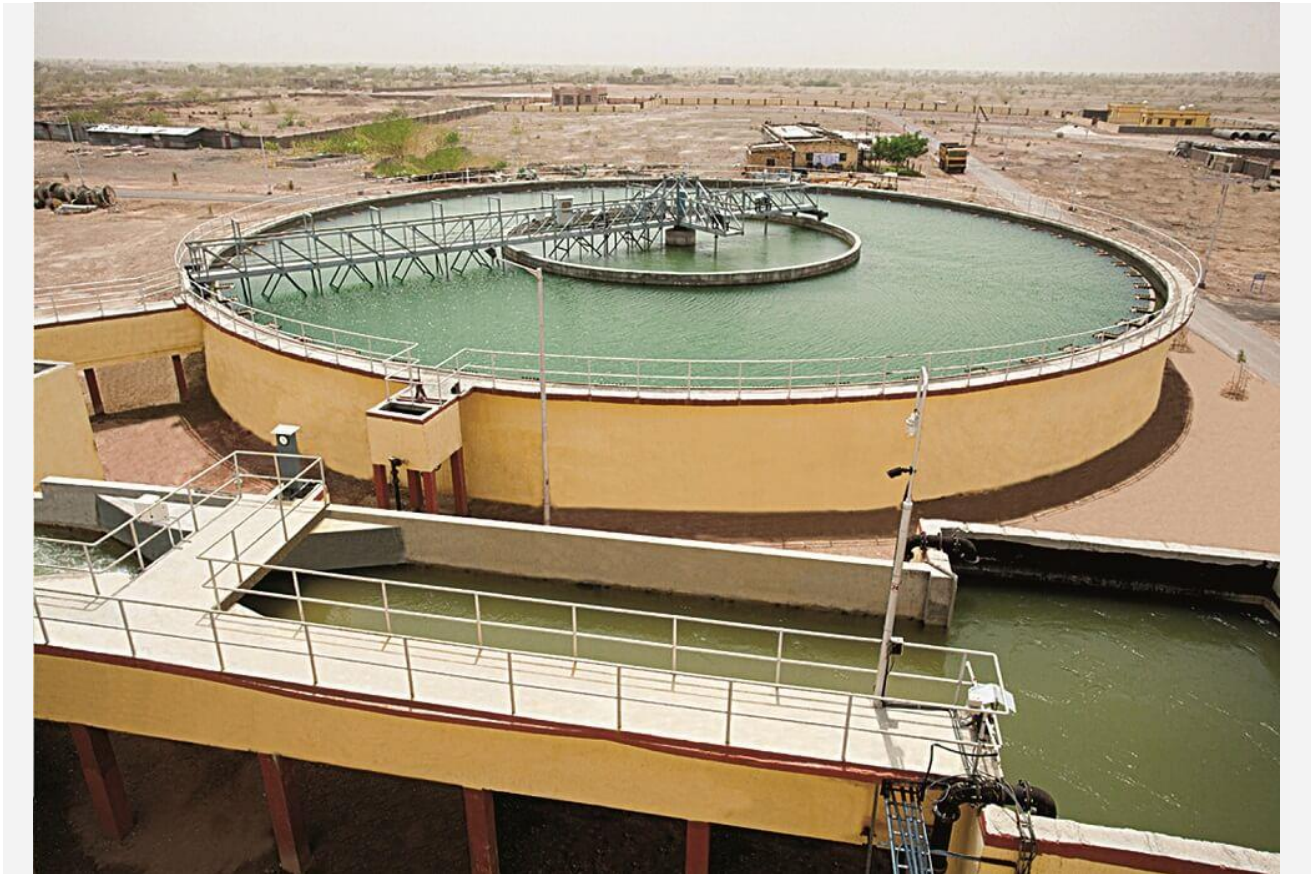
125 MLD Water Treatment Plant at Pokhran
