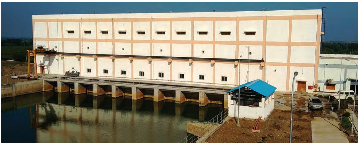
2587 MLD Pumping House for SAUNI Yojana Phase-1, Gujarat
