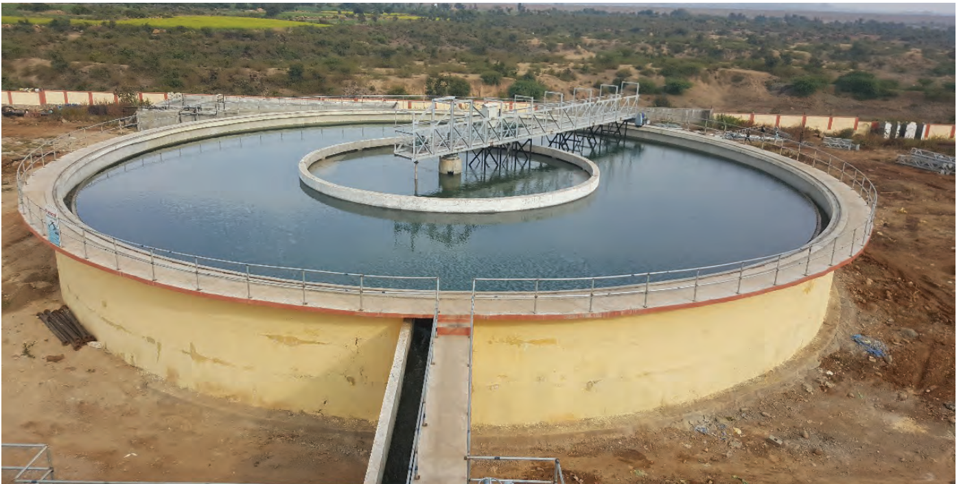
19 MLD Water Treatment Plant, Gagreen
