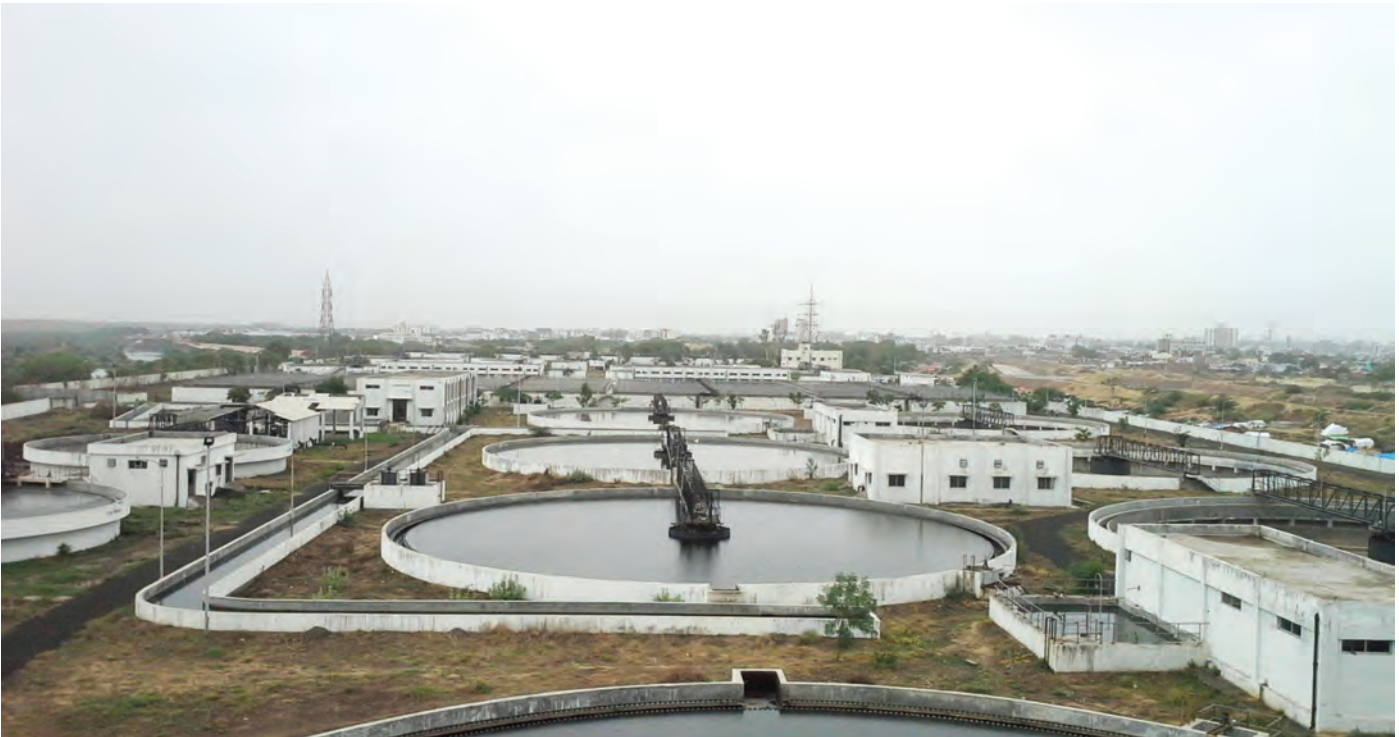
240 MLD STP at Ahmedabad, Gujarat
