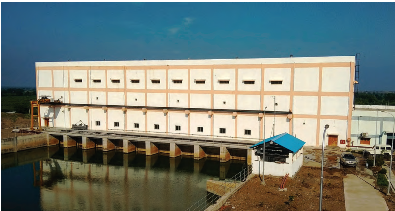
2587 MLD Pumping House for SAUNI Yojana Phase-1, Gujarat
