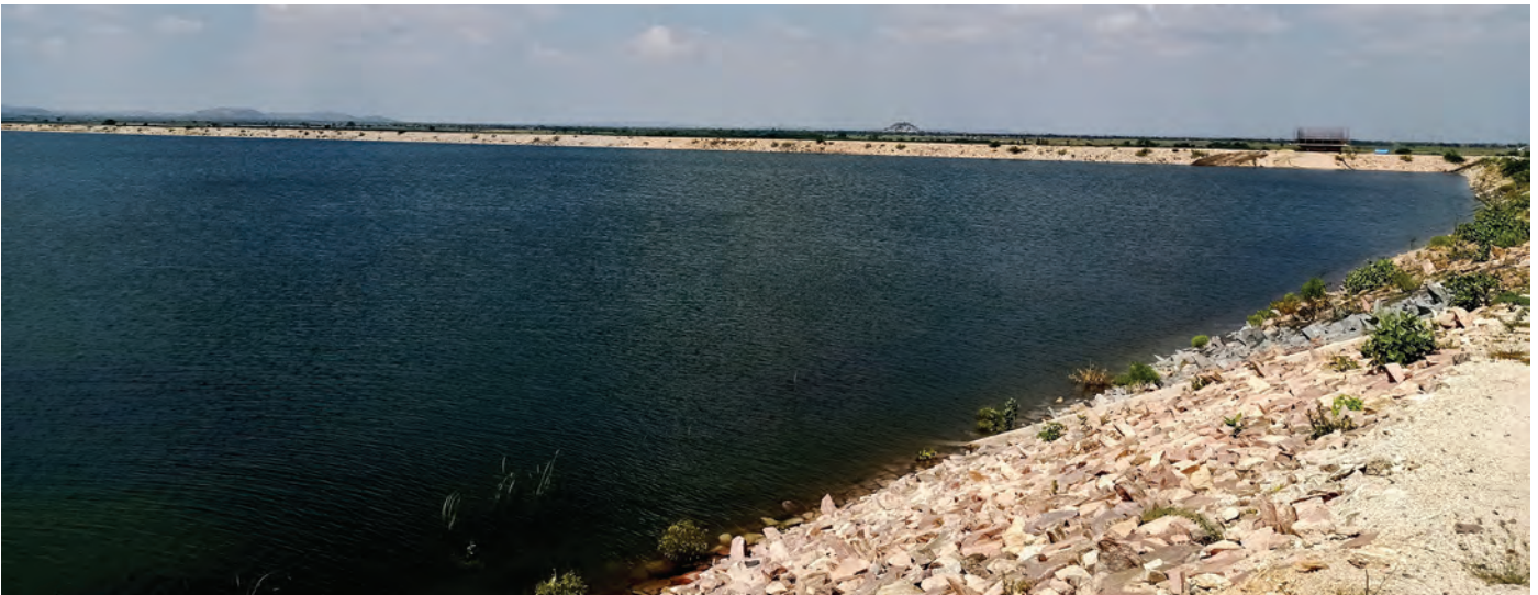
2074 Million Litre Raw Water Reservoir, Sindhanur, Karnataka
