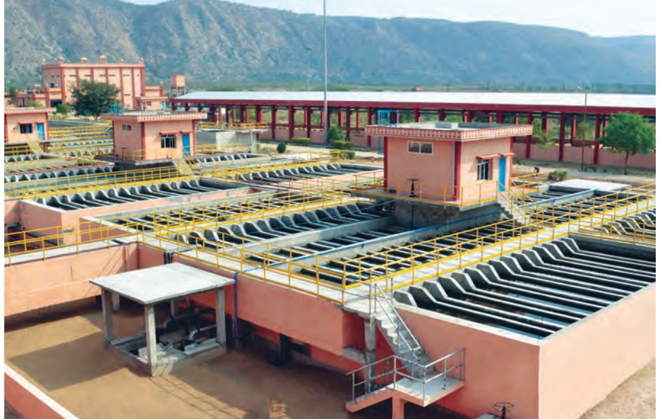
200 MLD Water Treatment Plant, Surajpura, Rajasthan
