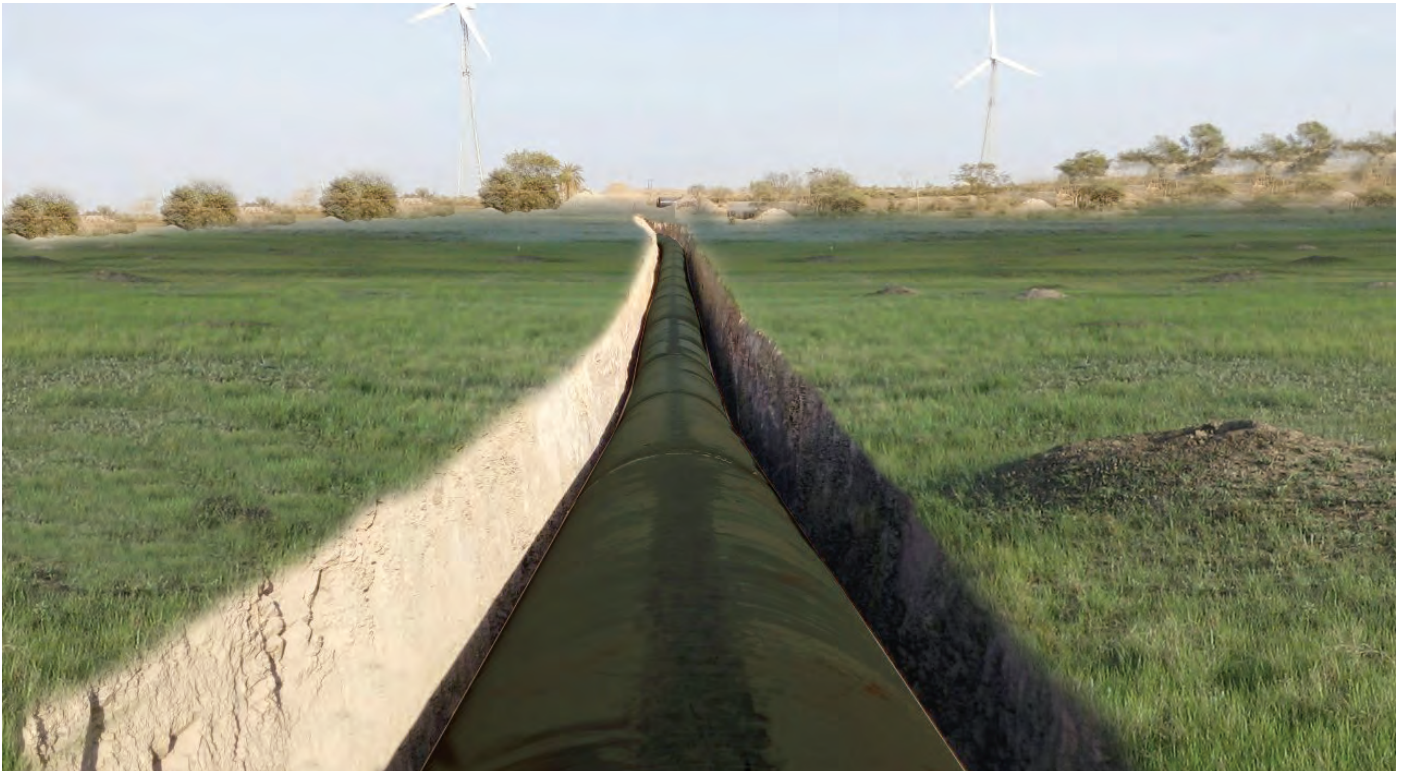
3000 MM Dia MS Sauni Pipeline, Gujarat
