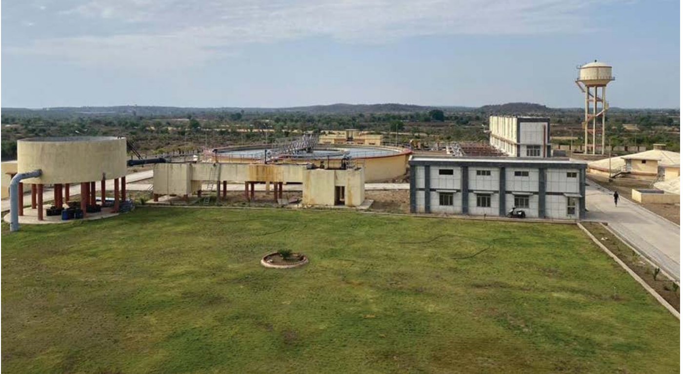
Gagreen Water Supply Scheme, Rajasthan
