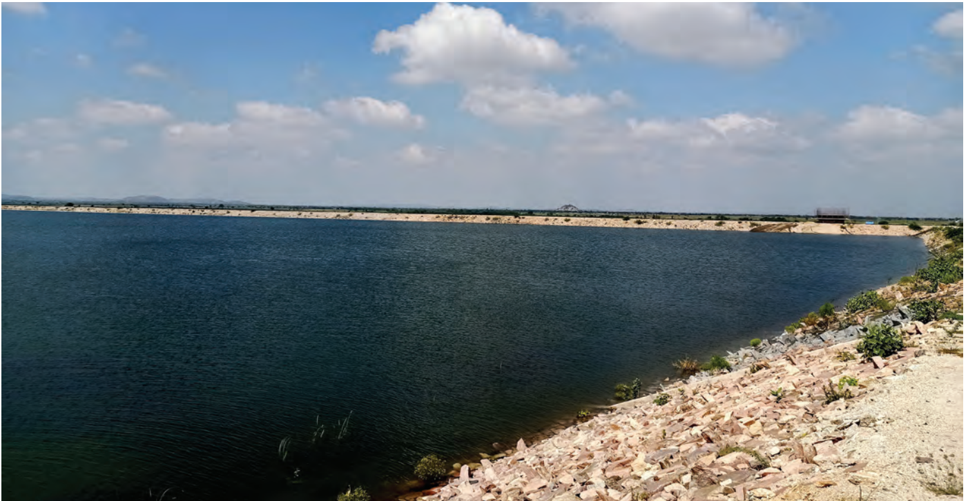
2074 Million Litre Raw Water Reservoir, Sindhanur, Karnataka
