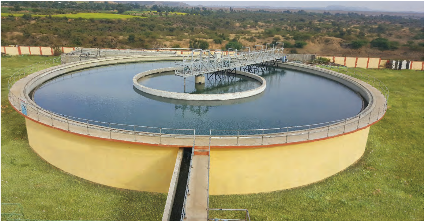
19 MLD Water Treatment Plant, Gagreen, Rajasthan
