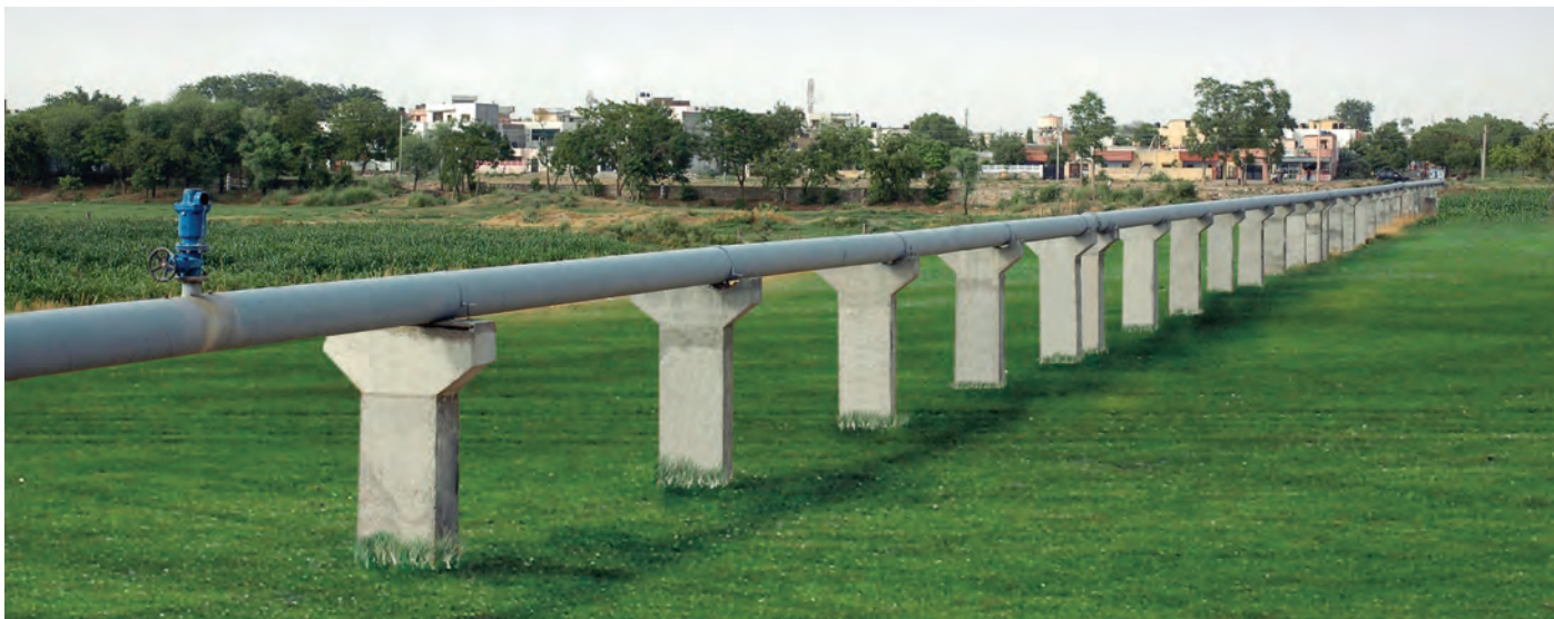
Bisalpur Jaipur Water Supply Pipeline
