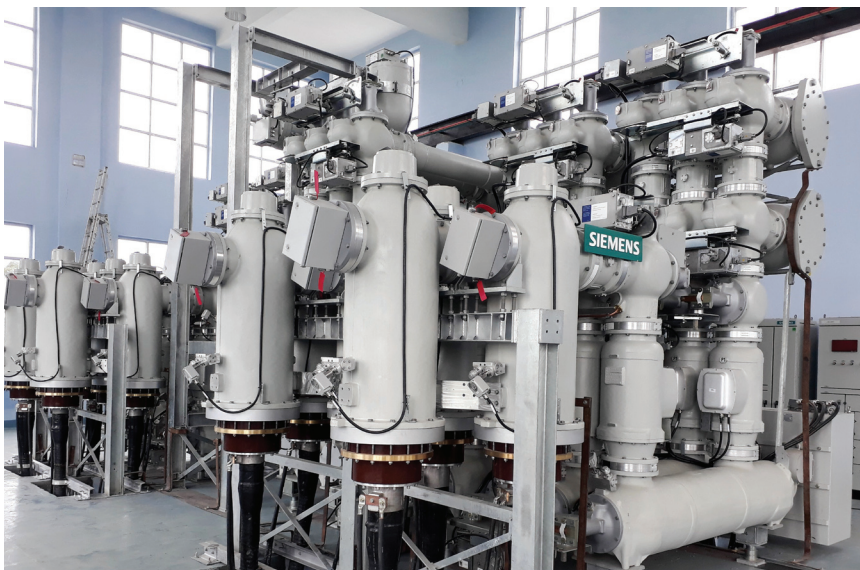
220kV GIS substation, Alipurduar, West Bengal
