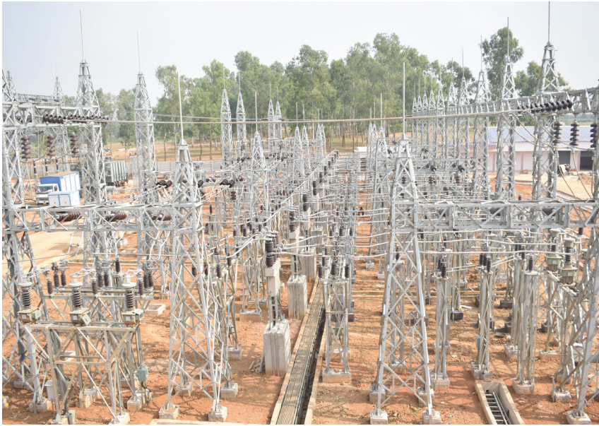
220kV AIS substation, Ratu, Jharkhand
