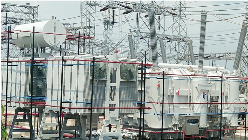
500 MVA auto transformer, Mainpuri, Uttar Pradesh
