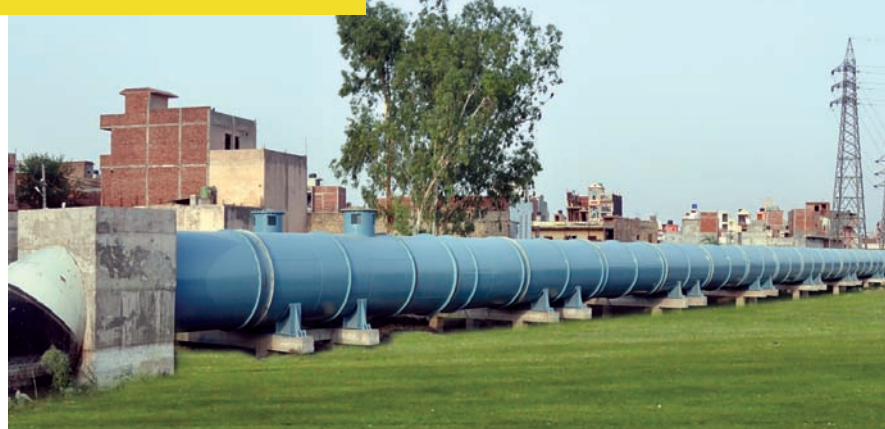
2420 MM MS PIPELINE FOR BULK WATER SUPPLY IN DELHI
