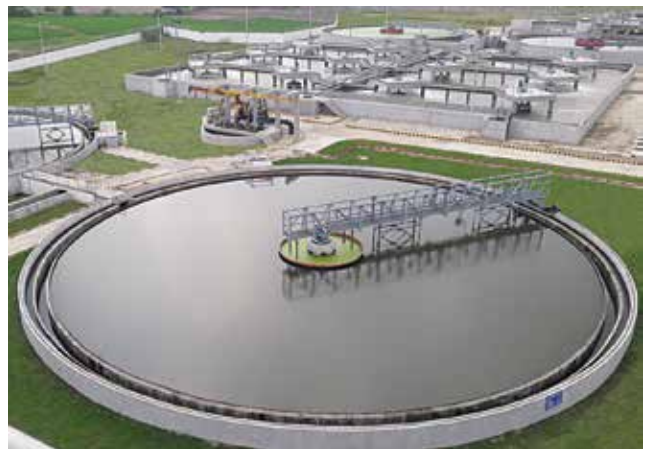
42 MLD Sewage Treatment Plant, Kanpur
