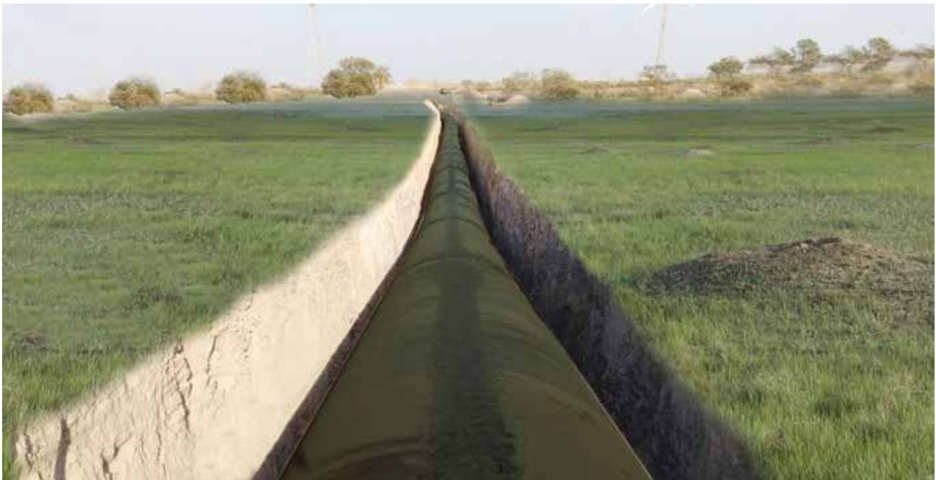
3000 MM Dia MS Sauni Pipeline, Gujarat
