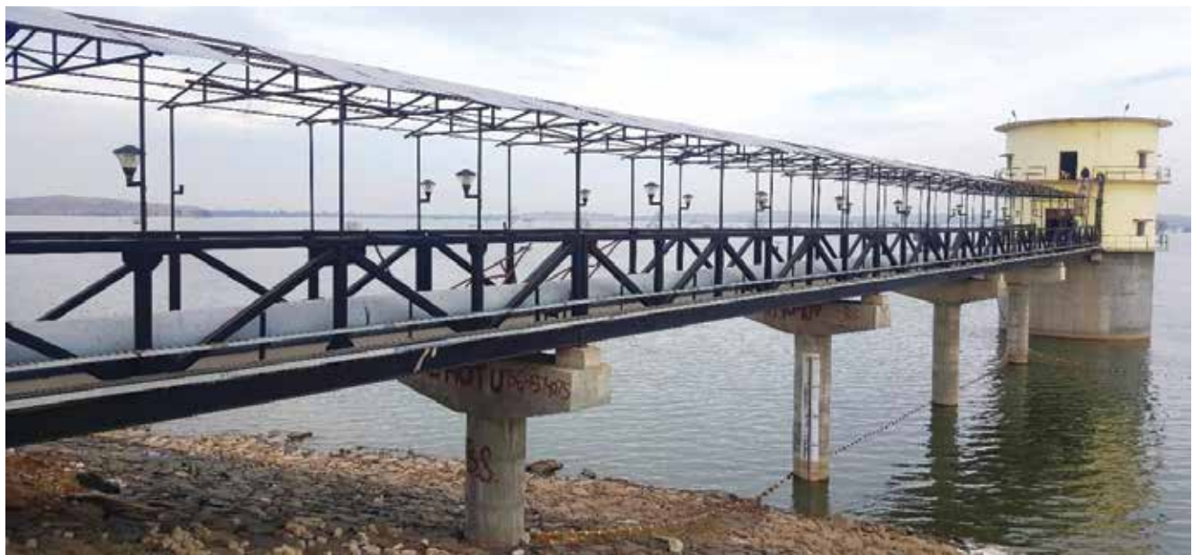
Water Intake at Gagreen Dam, Rajasthan
