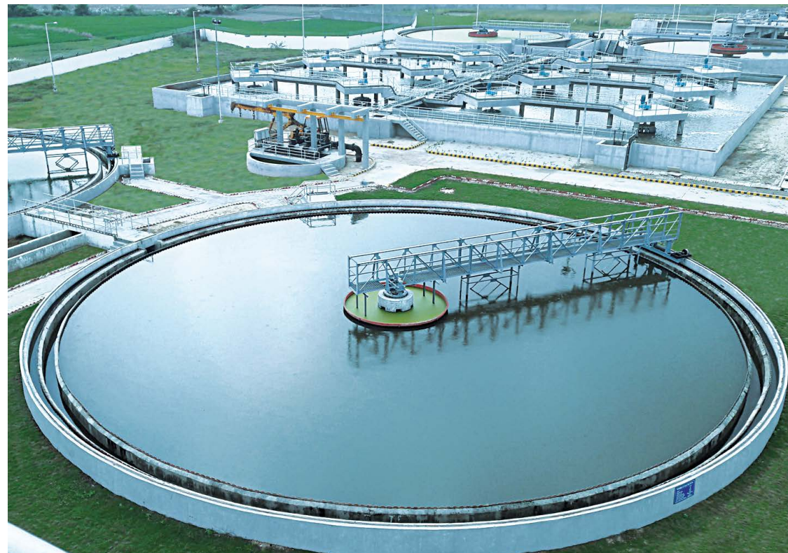
42 MLD Sewage Treatment Plant, Kanpur
