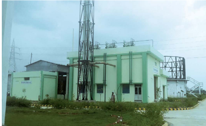
Gas Holder at 42 MLD STP, Kanpur
