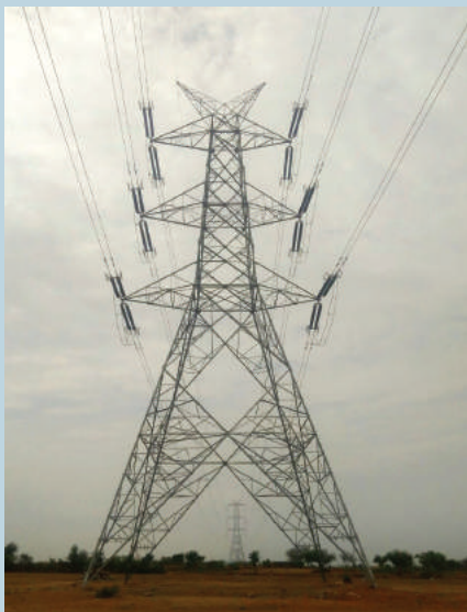
400 kV DC twin-moose transmission line from Chittorgarh to Bhilwara in Rajasthan. Project contractor and source of photograph: SPML Infra Ltd
