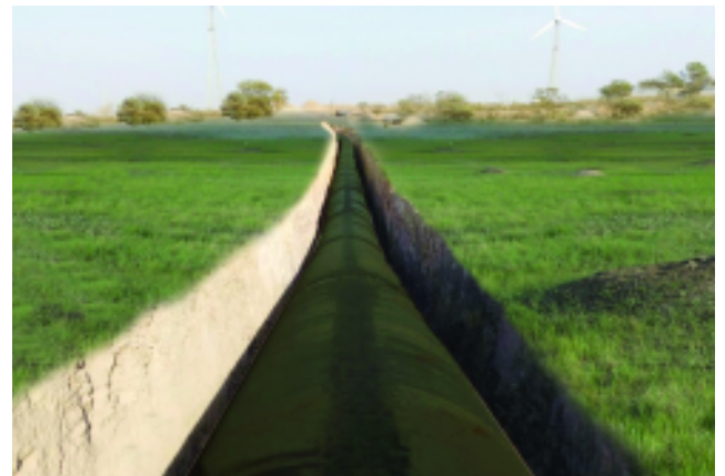
3000 MM Dia MS Sauni Pipeline, Gujarat
