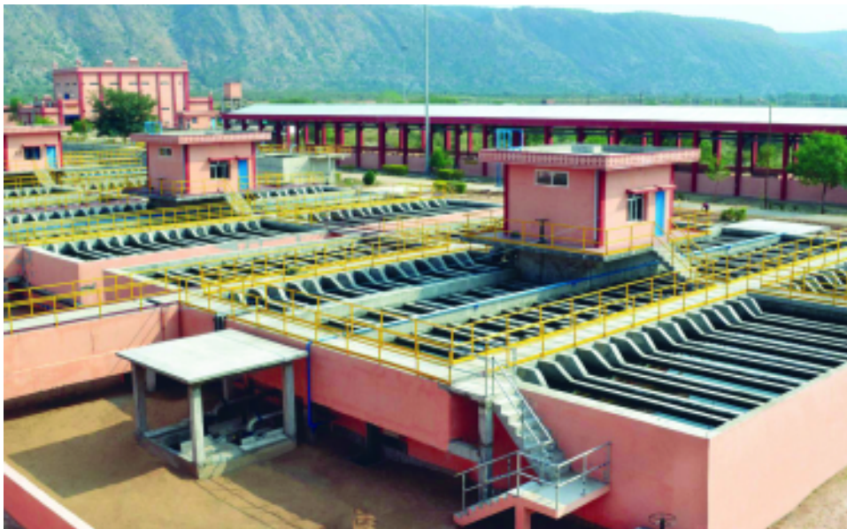
200 MLD Water Treatment Plant, Surajpura, Rajasthan
