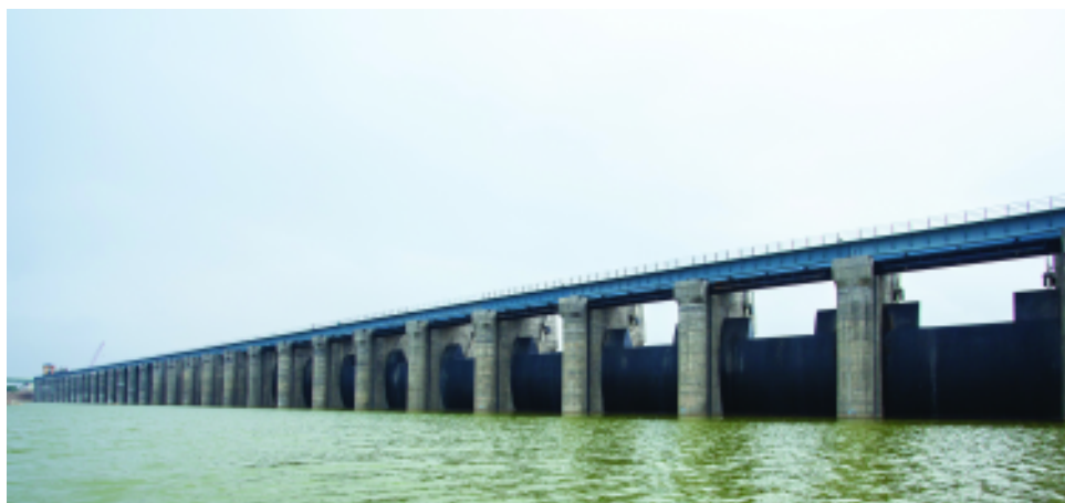
Kalisindh Concrete Gravity Dam, Rajasthan
