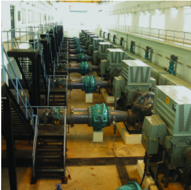
500 MLD Water Pumping Station, Bangalore
