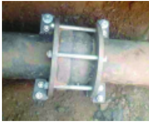
Mechanical Joint in Supply Pipeline in Bengaluru NRW Project
