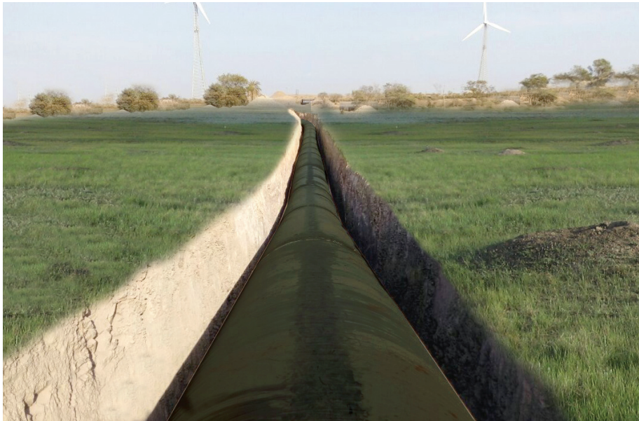
3000 MM Dia MS Sauni Pipeline, Gujarat
