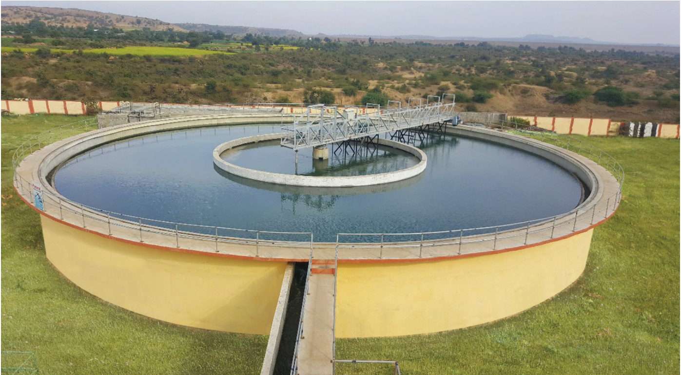
19 MLD Water Treatment Plant, Gagreen, Rajasthan
