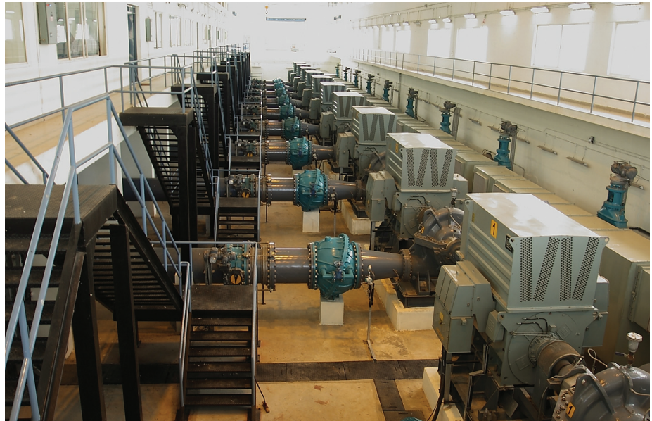
500 MLD Water Pumping Station, Bangalore
