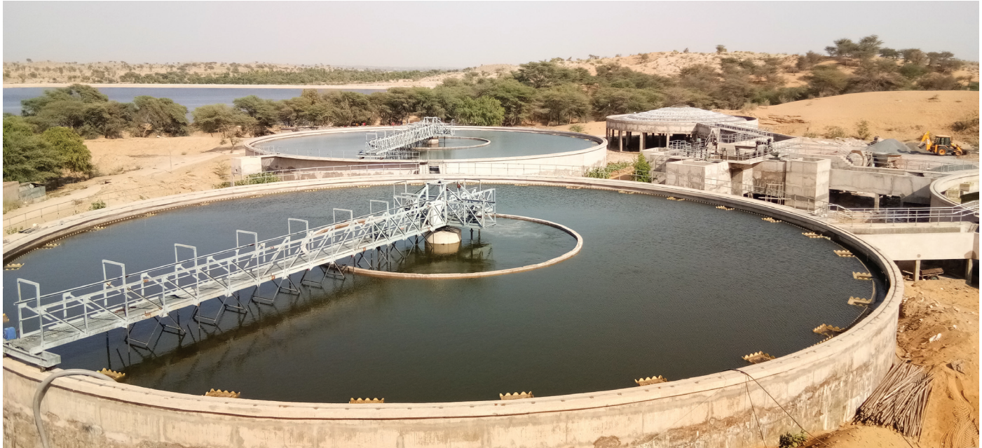
160 MLD Water Treatment Plant, Dhannaser, Rajasthan
