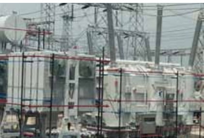
500 MVA Autotransformer, Mainpuri, Uttar Pradesh
