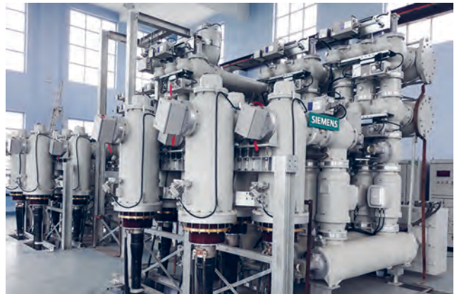
220 kV GIS Substation, Alipurduar, West Bengal
