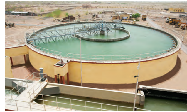
125 MLD Water Treatment Plant at Pokhran
