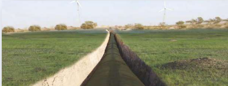
3000 MM Dia MS Pipeline, Sauni Yojana, Gujarat
