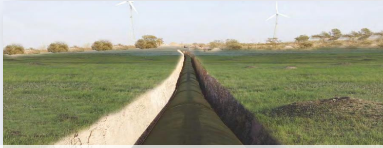
3000 MM Dia MS Pipeline, Sauni Yojana, Gujarat
