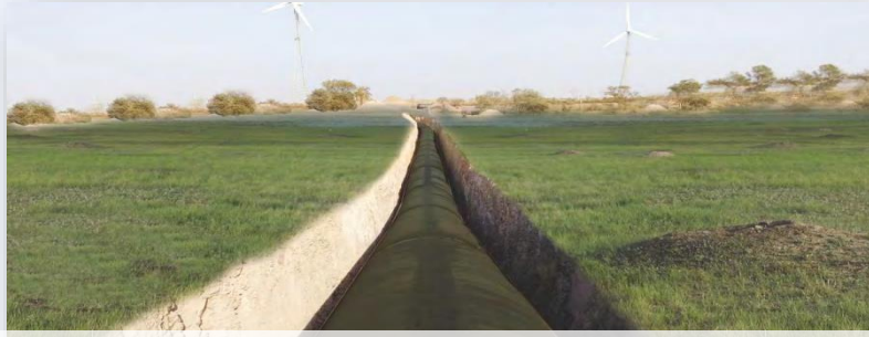
3000 MM Dia MS Pipeline, Sauni Yojana, Gujarat
