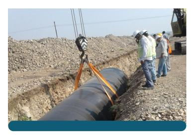
Gujarat. The pipe laying work for 36.6 kms MS Pipeline of 3000 mm diameter of 17.5 mm thickness with external 3LPE coating & internal food grade epoxy coating has begun under the Link 1, Package IV as part of the Phase II of Saurashtra-Narmada Avtaran Irrigation Yojana.
