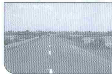
A state highway in Madhya Pradesh. Photo: MPRDC Ltd
