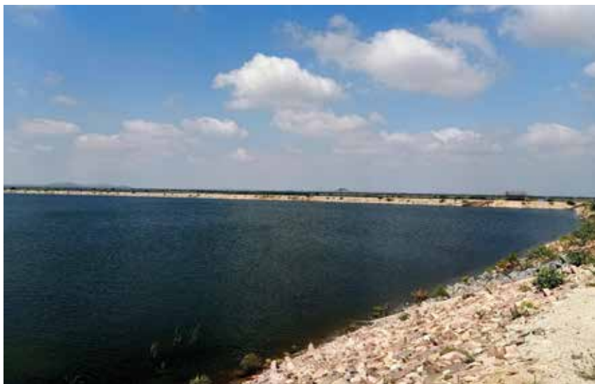
2074 Million Litre Raw Water Reservoir, Sindhanur, Karnataka
