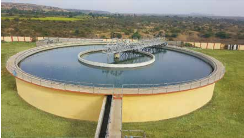
19 MLD Water Treatment Plant, Gagreen
