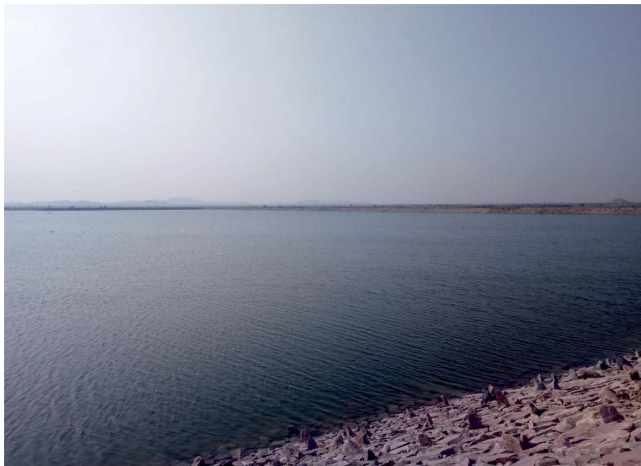
2074 Million Litres Raw Water Reservoir, Sindhanur, Karnataka
