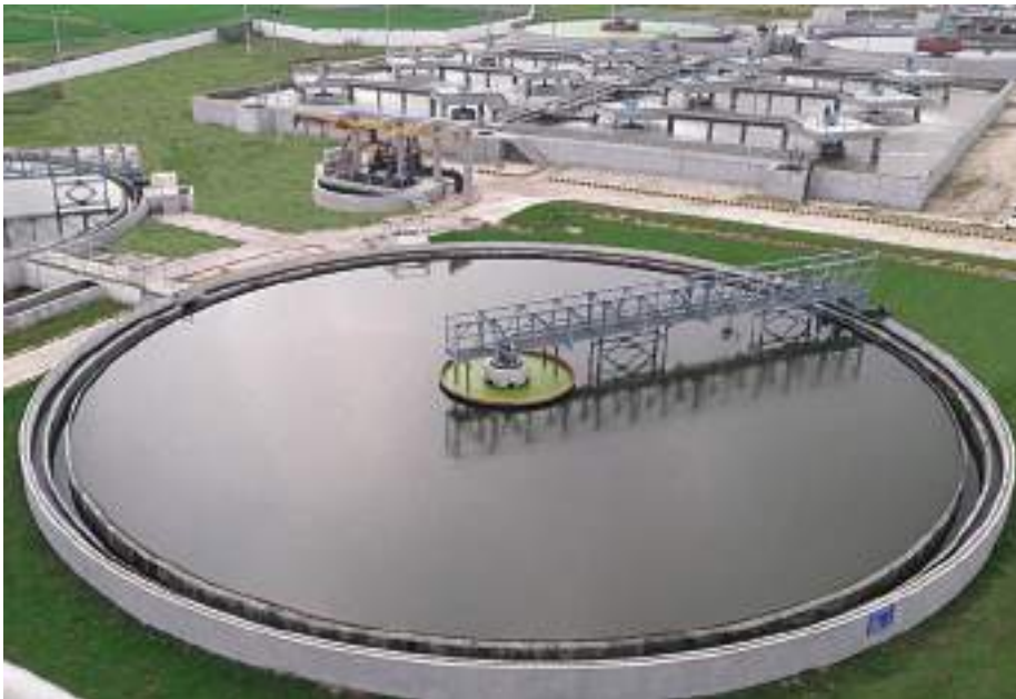
42 MLD Sewage Treatment Plant, Kanpur
