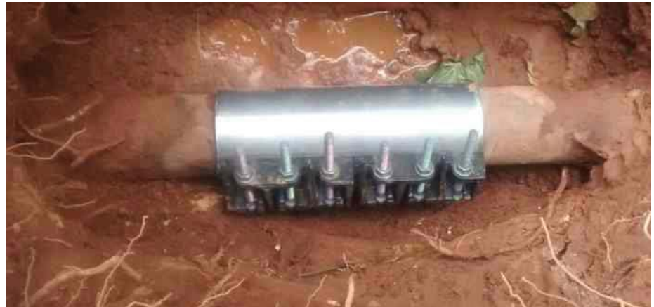
Split collar to repair barrel crack in Bengaluru NRW Project
