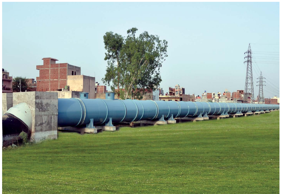
2420 MM MS Pipeline for Bulk Water Supply in Delhi
