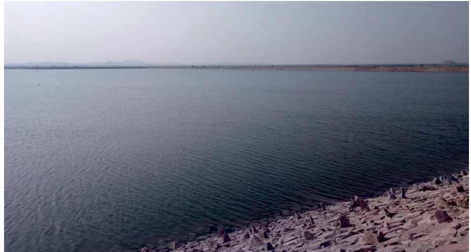
2074 Million Litres Raw Water Reservoir, Sindhanur, Karnataka
