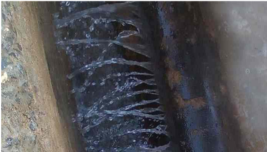
Damaged supply line in Bengaluru
