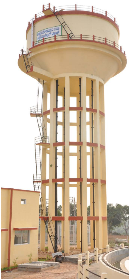
Honsur Water Reservoir, Karnataka
