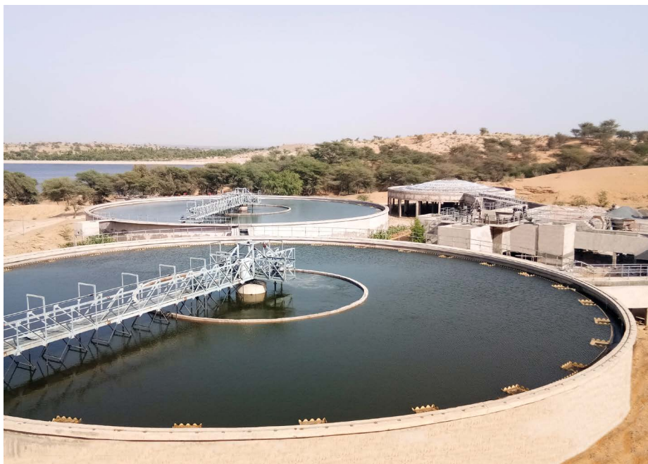
160 MLD Water Treatment Plant, Dhannaser, Rajasthan
