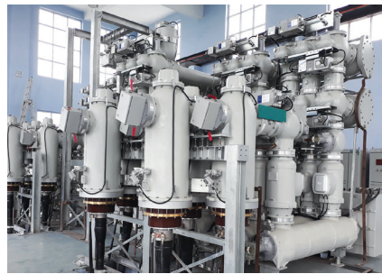
220kV GIS Substation, Alipurduar, West Bengal
