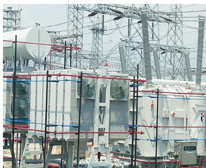
500 MVA Autotransformer, Mainpuri, Uttar Pradesh
