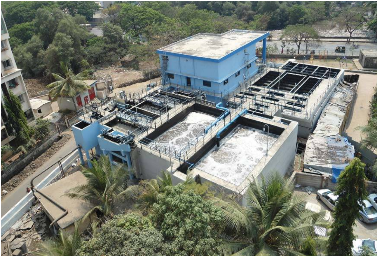
13 MLD Sewage Treatment Plant in Zone 6 in Mira Bhayandar
