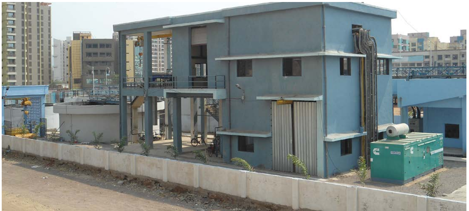
17 MLD STP at Zone 5 in Mira Bhayandar
