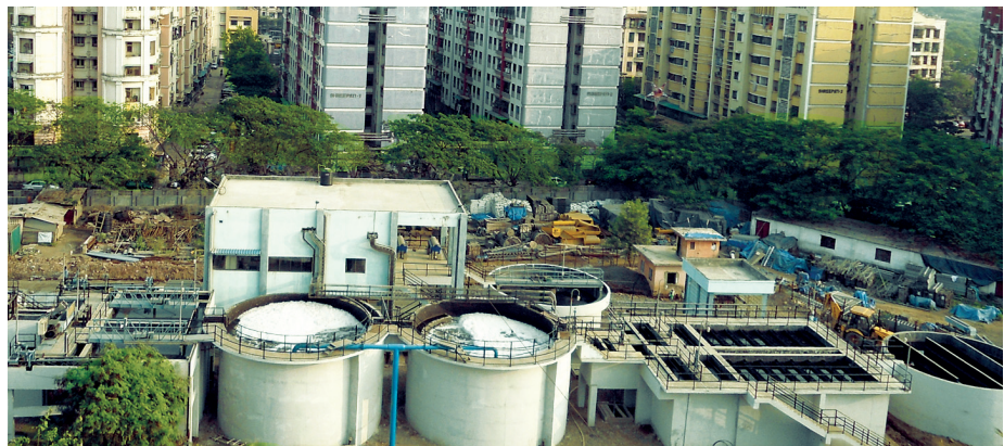
11 MLD Decentralized Sewage Treatment Plant at Mira Bhayander
