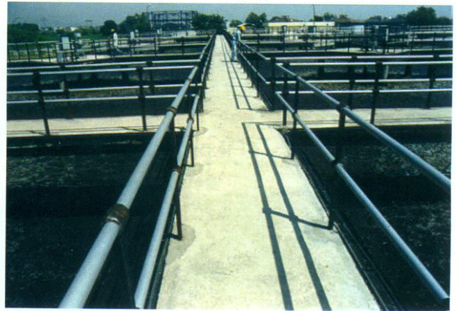
Sewage Treatment Plant, Okhla, Delhi
