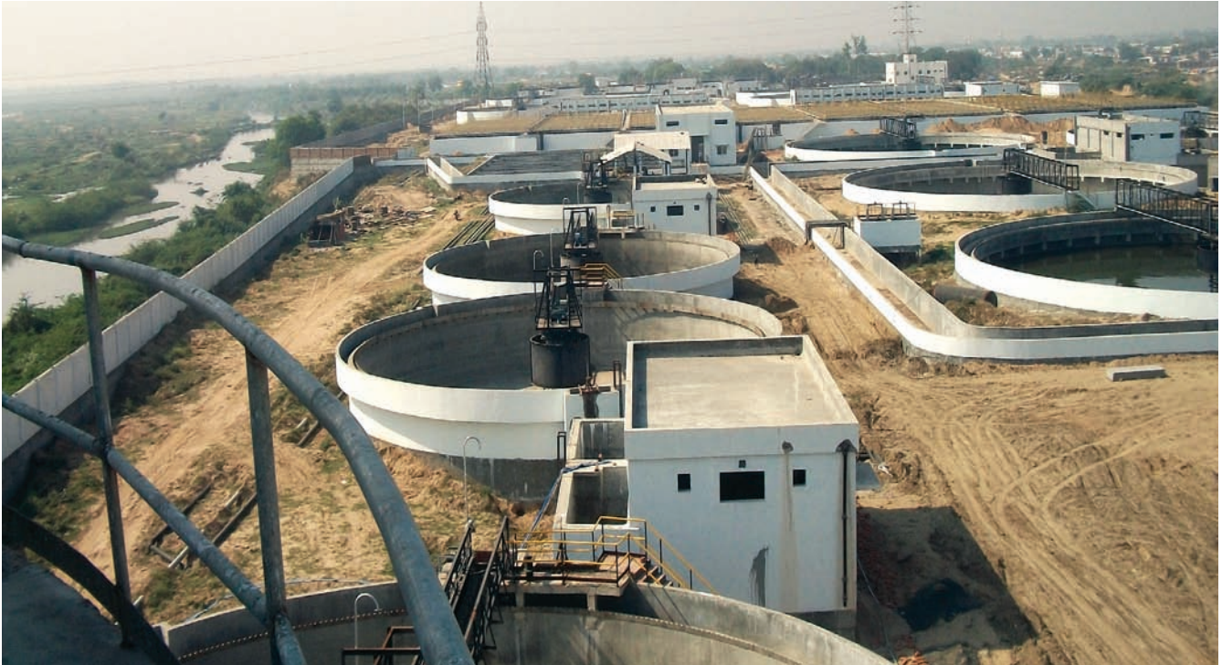
Aerial view of the 240 MLD sewage treatment plant at Ahmedabad, Gujarat, built by SPML
