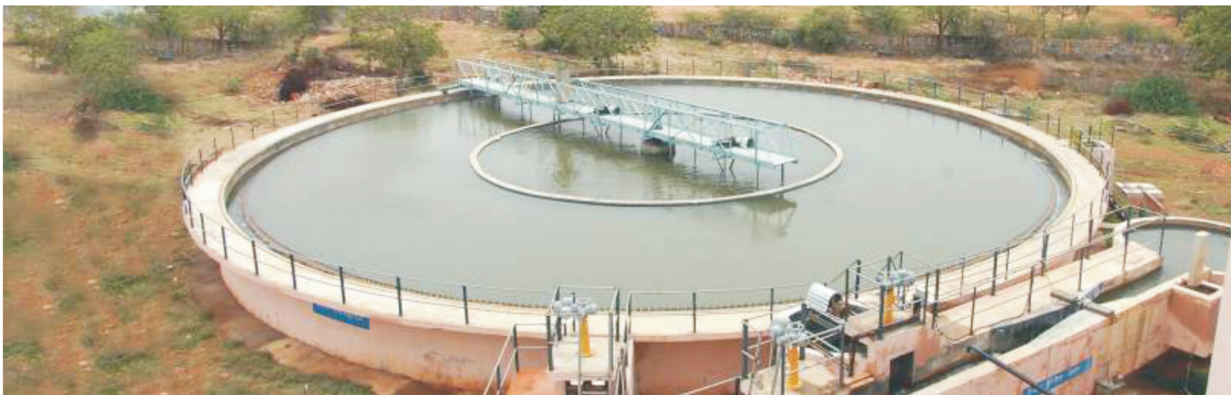
19.5 MLD water treatment plant at Ramganjmandi, Rajasthan
