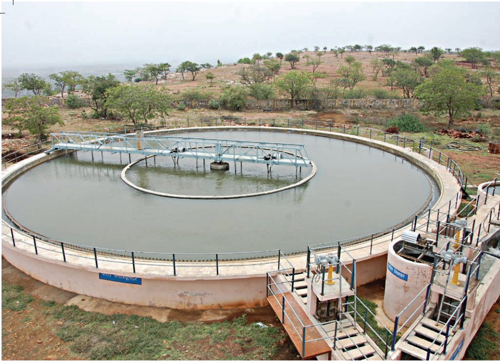
Ramganjmandi Water Treatment Plant
