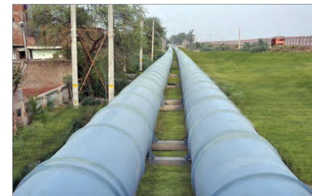
2420 MM dia twin Water Pipeline at Wazirabad, Delhi
