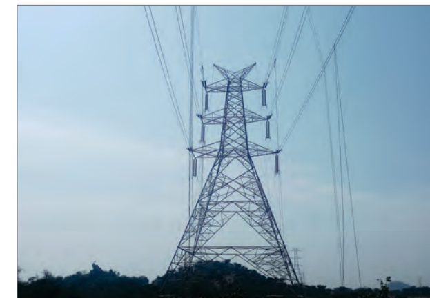
400 kV Twin Moose Transmission Line, Bhilwara, Rajasthan
