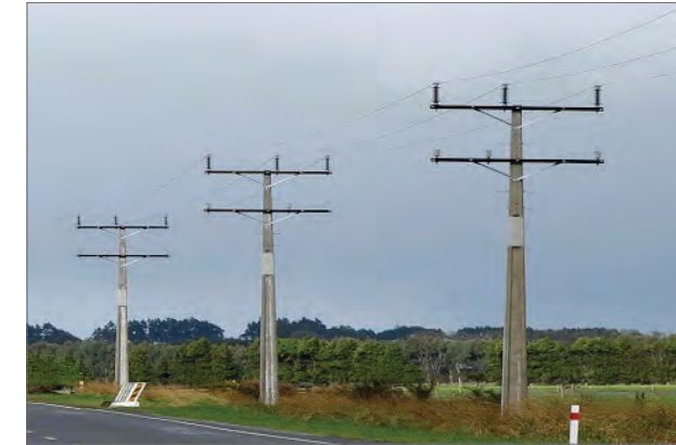
11 kV Feeder Separation Line, Jabalpur, Madhya Pradesh
