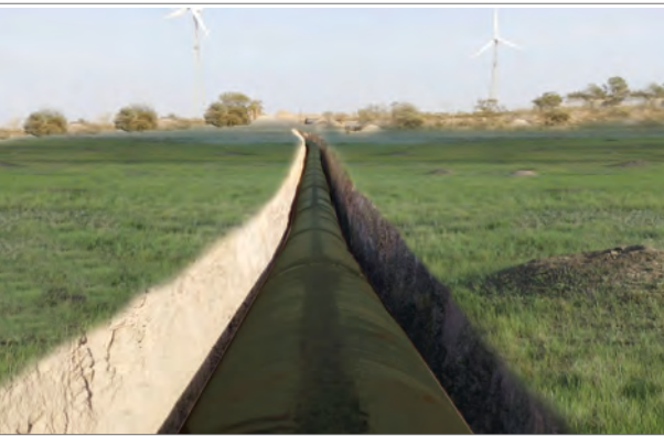
3000 MM Dia MS Pipeline, Sauni Yojana, Gujarat
