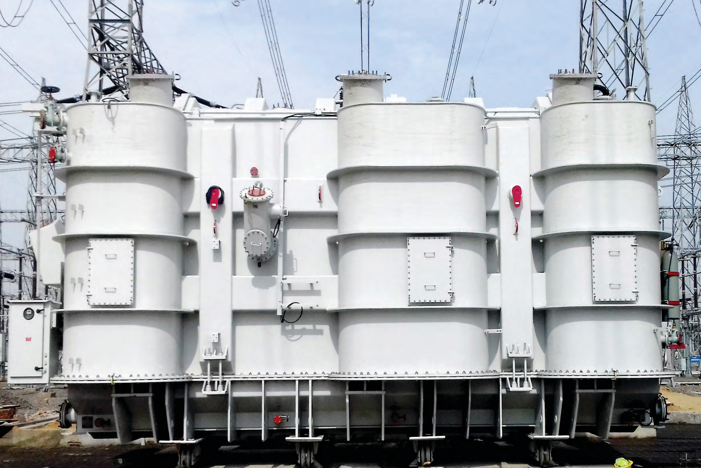
500 MVA Autotransformer, Sikar, Rajasthan
