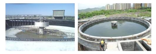
stabilization of sludge. Stabilized and digested sludge will then be taken to mechanical dewatering system for dewatering of the sludge. Filtrate shall be taken back in to the system for treatment and dried sludge cake shall be
