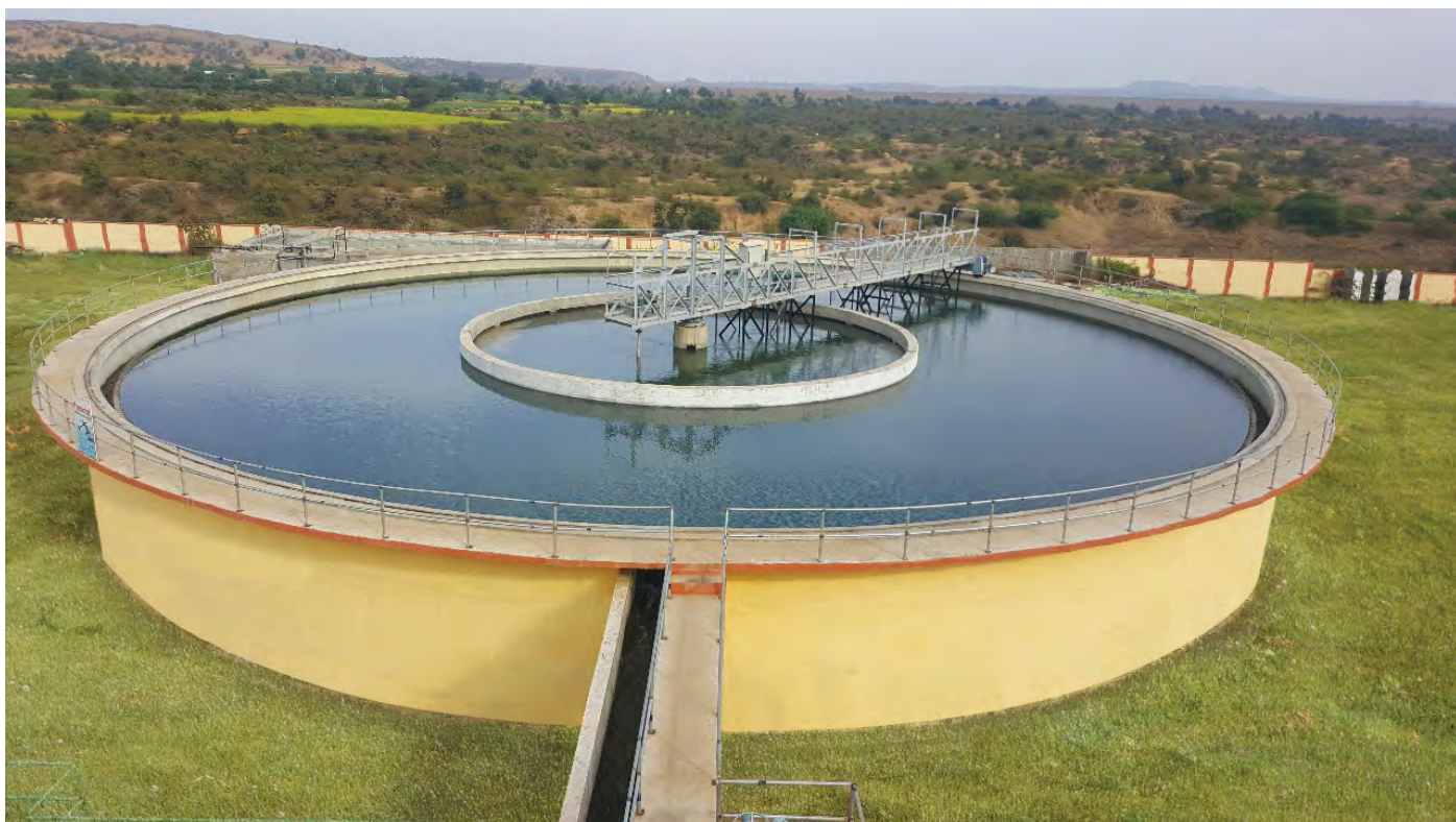
Water Treatment Plant, Gagreen, Rajasthan
