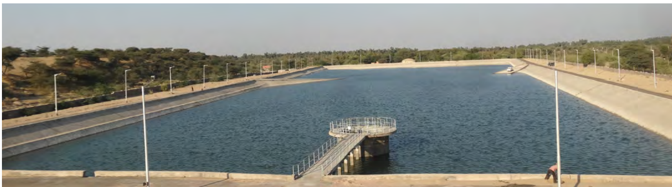
300 Million Litre Raw Water Reservoir at Pokhran, Rajasthan
