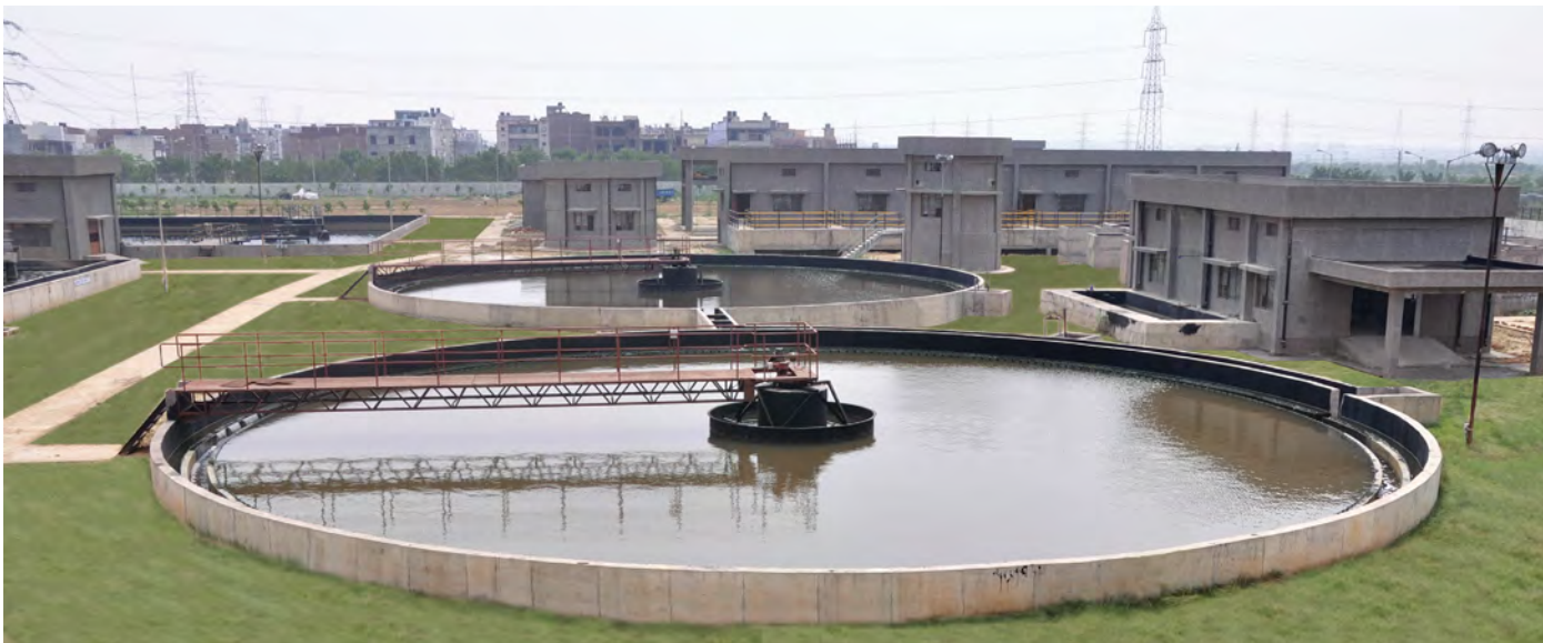
Industrial Wastewater Treatment Plant, Bawana, Delhi
