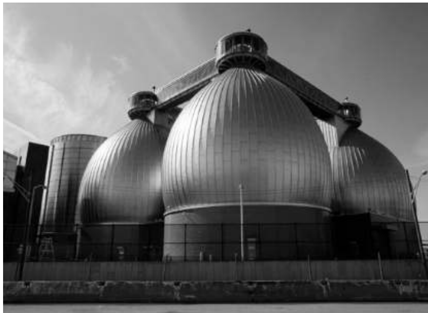
Fig 2.9 Anaerobic Treatment System
