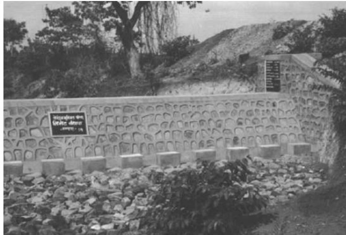
Fig 3.8: Using Check Dams
