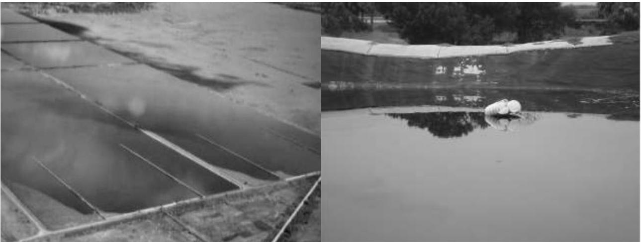
Fig 2.10 Waste stabilization ponds (WSPs)
