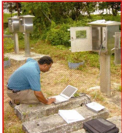
Water utility managers need to accurately measure water produced from the treatment facility. Total water produced is a key input for the water balance.
