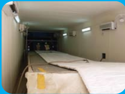
Wet Out Process In Progress
