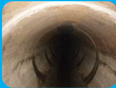
Desilted Jail Road Sewer
