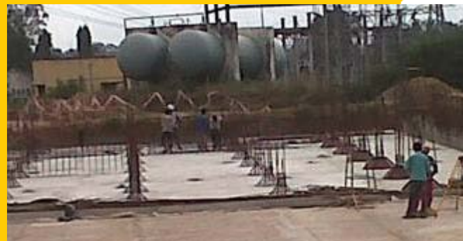
Harohalli pumphouse area raft-column base under construction
