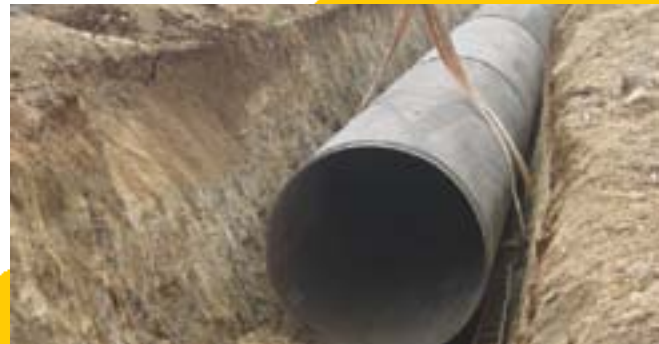
Laying of pipeline
