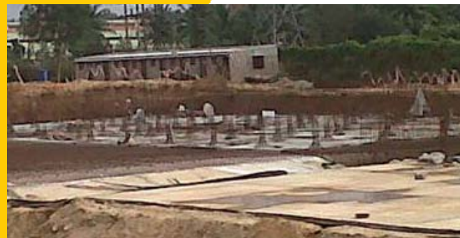
Harohalli Reservoir Area Raft and Column Bases under progress TK Halli
