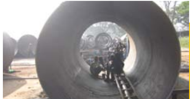
Guniting - Internal Coating
