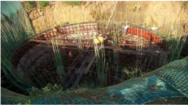
This photograph shows Sewage Pumping Station at Zone 7 at advance stage of completion. The work is being done by open excavation method as strata was good
