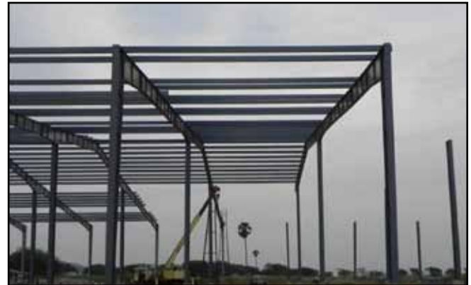
Monsoon Shed – Column Erection Complete, Rafter and Purlin Erection in Progress
