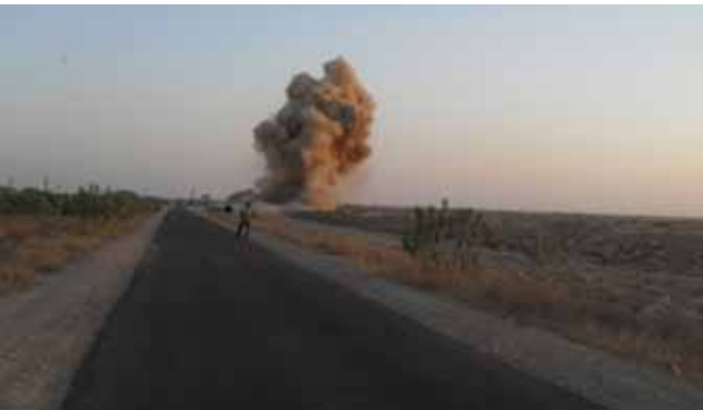
During Blasting process prohibited area is evacuated for any probable mishap.
