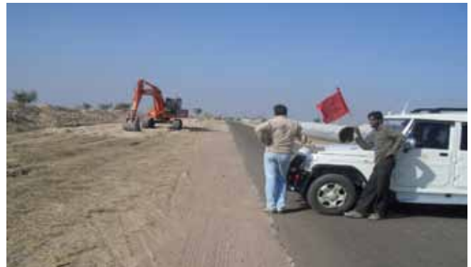
Signal System for traffic & people inside the prohibited area at both ends.
