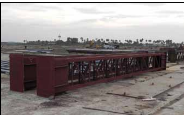
Refinement Area: Column Footings in Progress (60% Complete)
