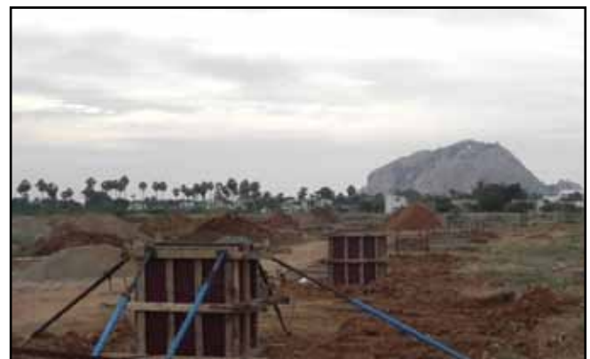
Refinement Area: Column Paint Work in Progress
