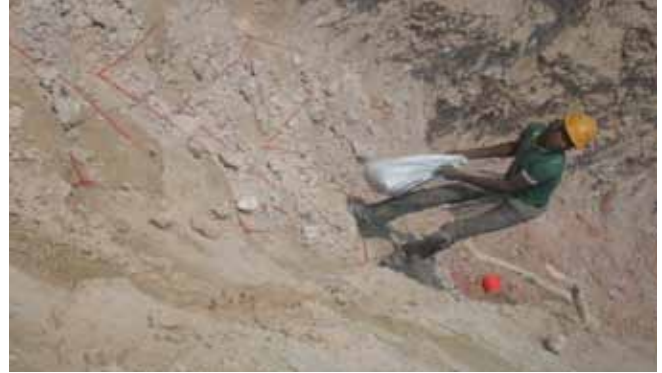
Wiring & filling of holes with explosives.
